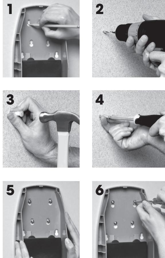
1. Using dispenser as a template, mark hole locations on wall. **(To be in compliance with ADA regulations, the dispenser should be mounted no more than 48" from the ground.) NOTE: Dispenser should be installed at least 6" above countertop.**
